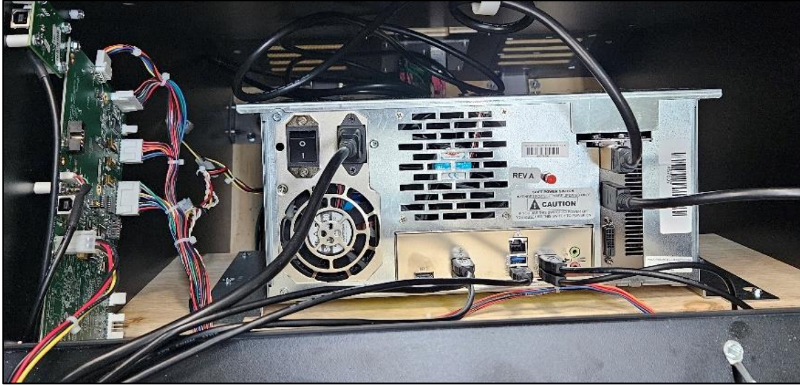
Final Connections with System Box Installed
