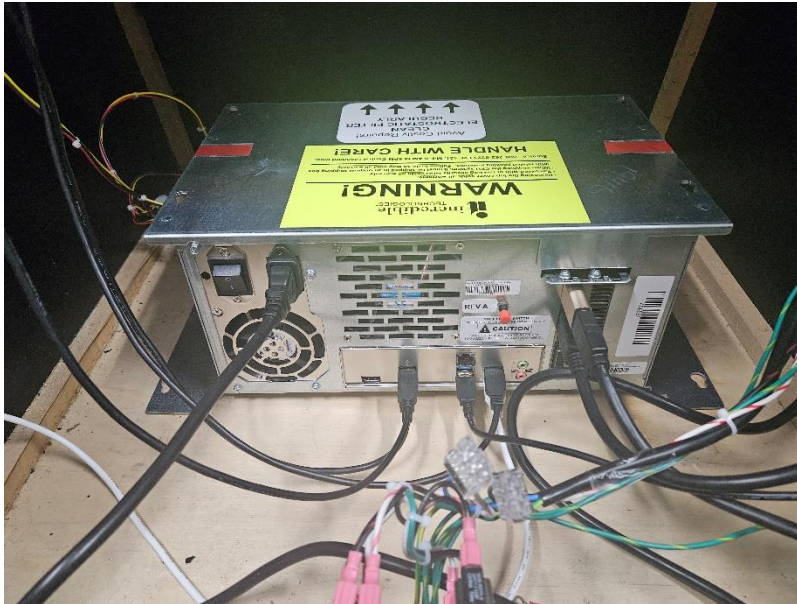
Final Connections with System Box Installed
